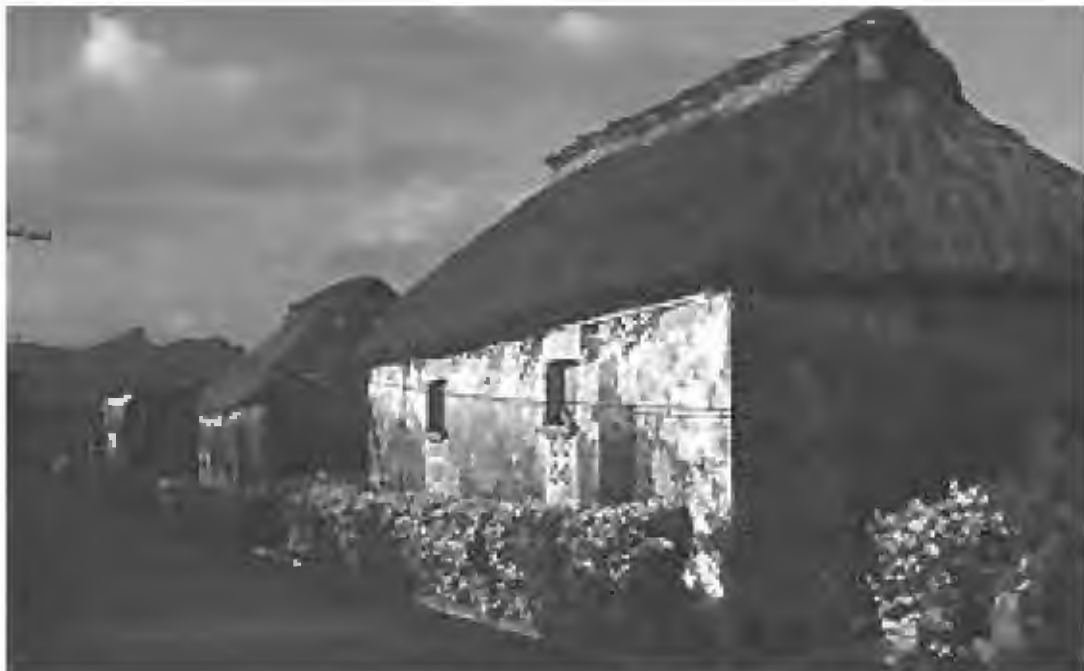
Figure 5. Houses in the province of Batanes, Philippines are made up of thick stone walls, and thick thatched roof for withstanding typhoons (Photo: Babiera, M; Source: Uy & Shaw; adapted from Hornedo, F., 2000; in UNISDR, 2008)
