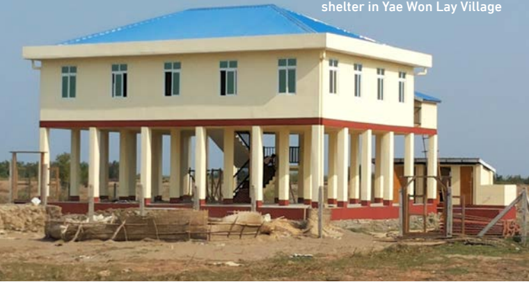
Figure 23. School/cyclone shelter in Yae Won Lay Village
