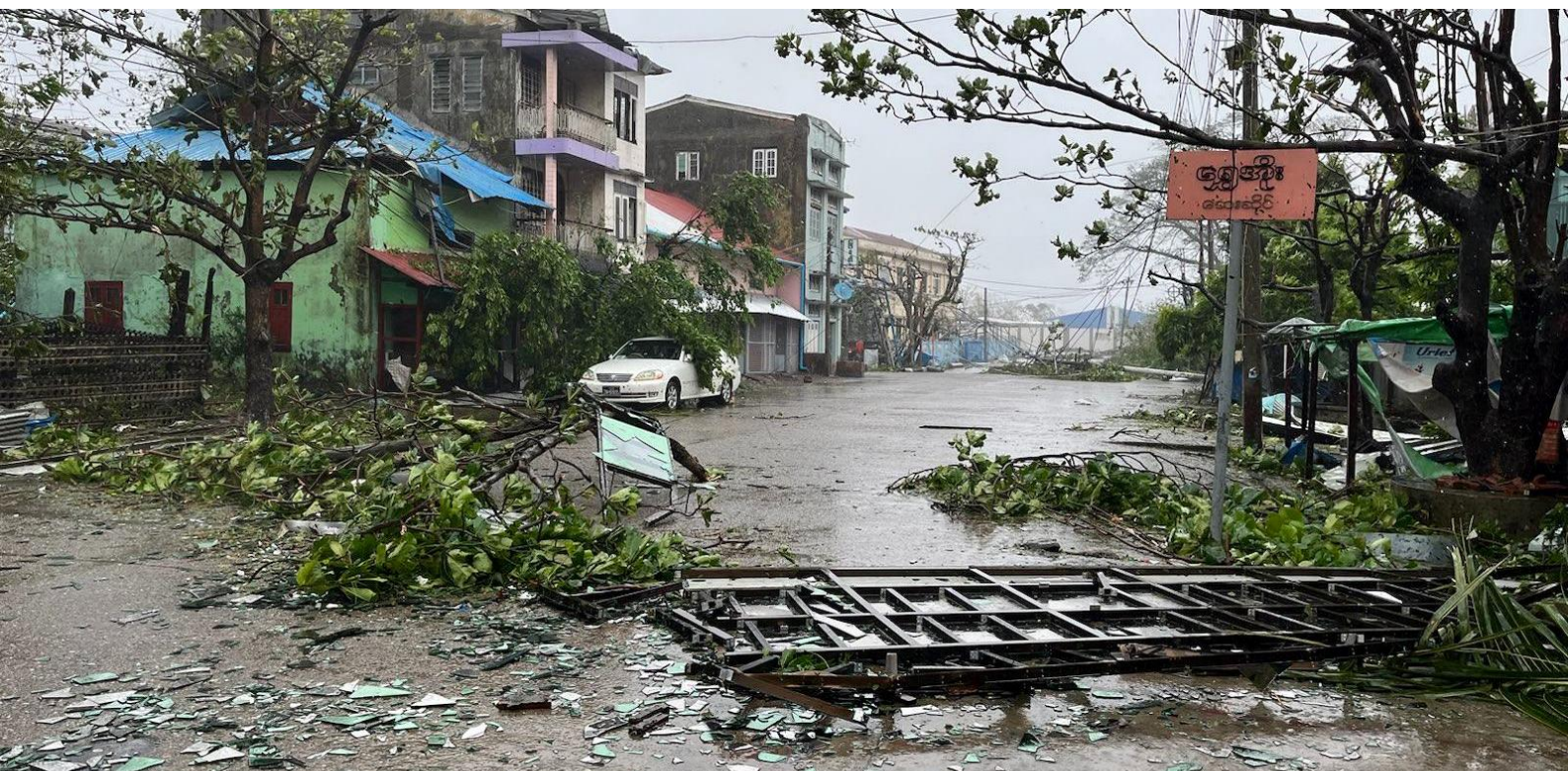
Destruction after Cyclone Mocha. Sittwe, Rakhine. Credit: UNOCHA/Suhad Sakalla/2023
