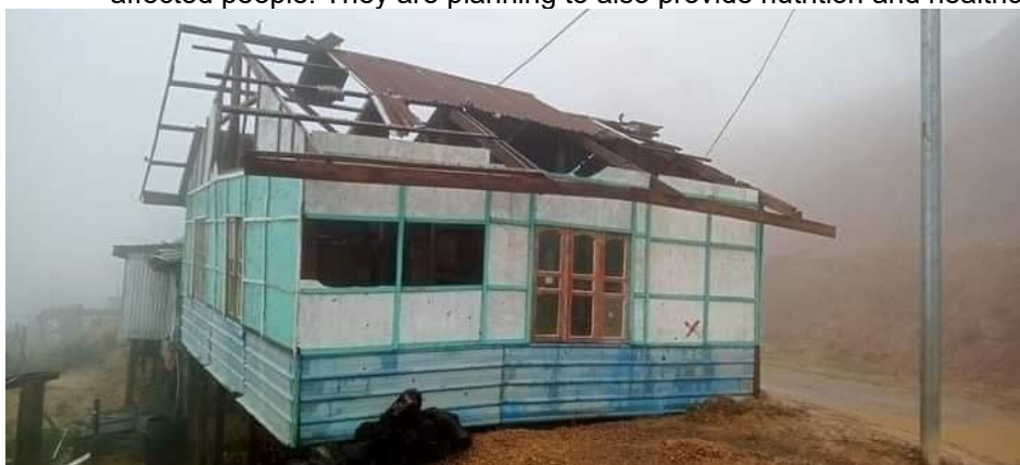
A house's roof ripped by Cyclone Mocha in Hakha township, Chin. Credit: Partner
