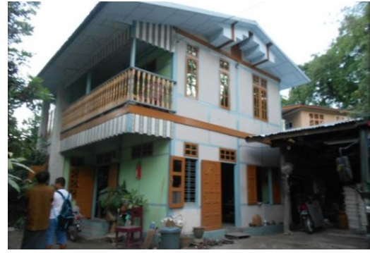
Figure (5) Brick Nogging Building Type
