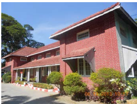
Figure (7) Brick Masonry Building Type
